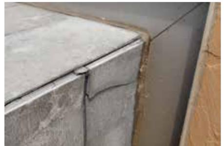
*Cracked grout due to missing transition movement joint.*
