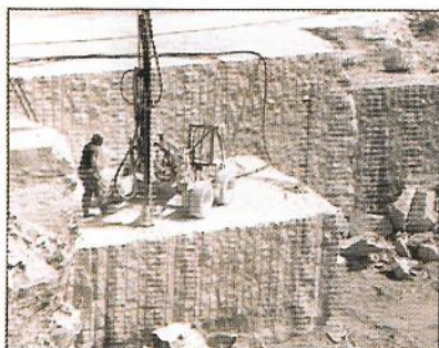
View of the Villebois Quarry (France) - Courtesy Euro-Marbles
