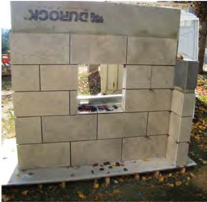
Mock-ups can serve as a critical component in the specification process. Pictured is an adhered veneer mock-up.
