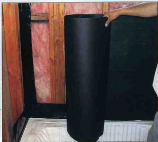
The photo at left illustrates the application of a moisture barrier over the flashing for a tub installation. At right, horizontal and vertical joints are properly caulked with a proper sealant.
