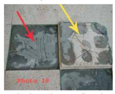
Spot-bonding is when an installer applies "spots" of adhesive on each corner of a tile and one in the center, and then presses it into place. This leaves voids under the tile, and ultimately throughout the entire installation, which can lead to big problems.
