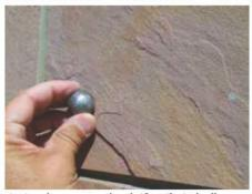
A simple way to check if a tile is hollow or solid sounding is to tap on the tiles with a hard object such as a steel ball bearing.
