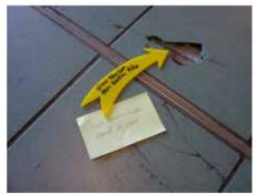
The lack of support beneath tile voids makes the tile more vulnerable to damage from live loads such as falling heavy objects, heavy equipment, rolling vehicles, loaded dollies, carts, etc.
