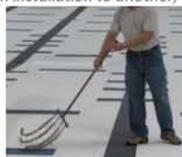
Notice if the hollow-sounding tiles are grouped together or are the spread out randomly — and is there pattern? Does the whole tile sound hollow or does only a portion of the tile sound hollow? In this instance, one also wonders about the solid-sounding tiles: do they have the same problem but haven’t debonded yet and might at a later date?
